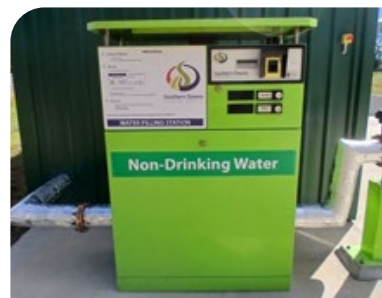
Mackenzie Street Standpipe
