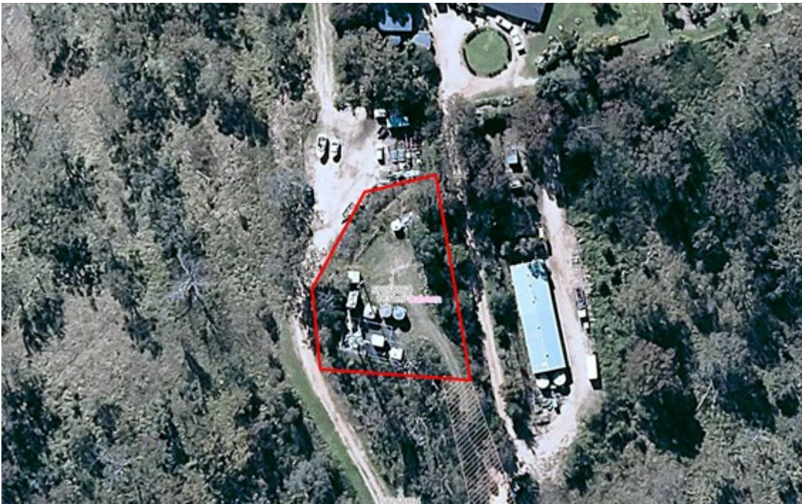
Figure 10: Aerial imagery of Telecommunications facility within Lot 1 SP268864
