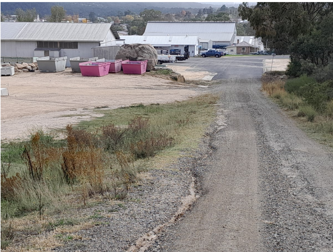
Figure 5: View looking north from the subject site. Note the impact of water runoff on the slope.
