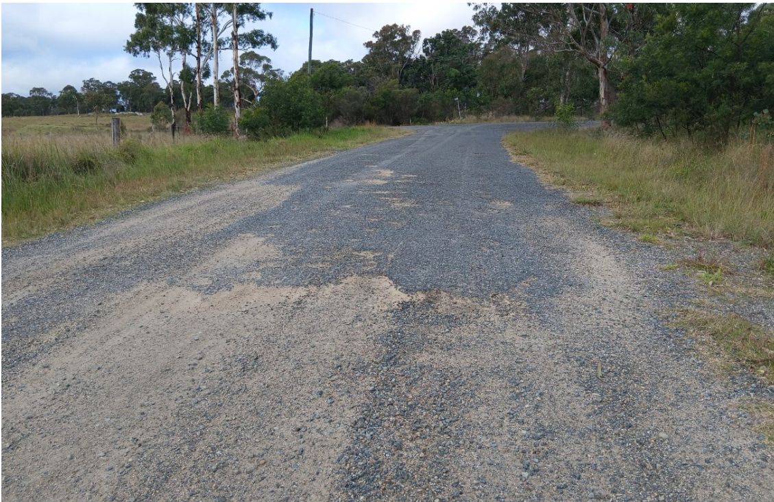
Photograph 1: Deutscher Road, transitioning from sealed to gravel construction
