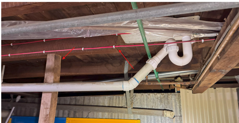
Figure 31 - Cut joists for pipework and inappropriate propping
