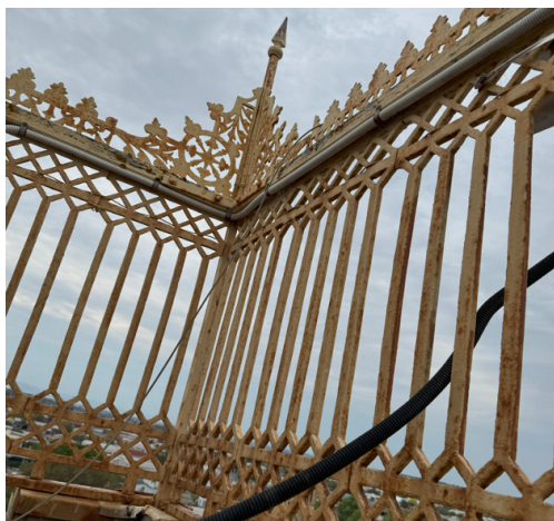
Figure 6 - Corrosion to balustrade and timber rot to rail
