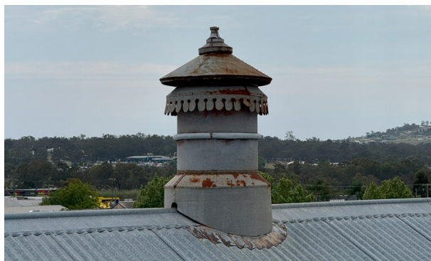
Figure 14 - Corrosion to ridge vents
