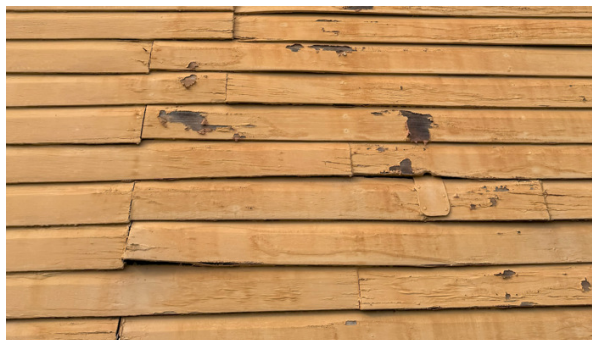
Figure 27 - Deteriorated weatherboards
