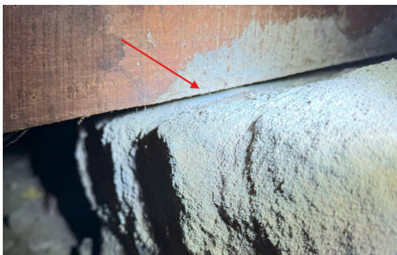
Figure 21 - Complete loss of grout pad
