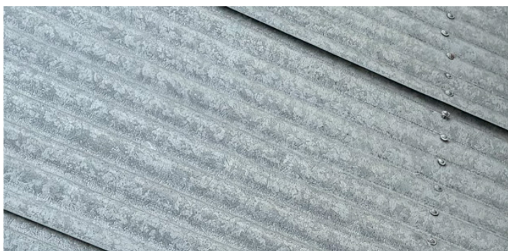
Figure 10 - Failed tiedown nails
