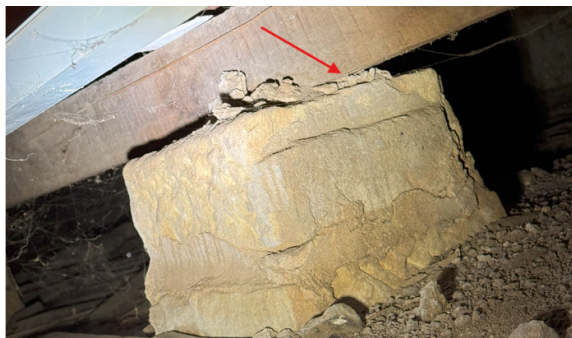
Figure 20 - Moderate deterioration and crumbling of grout pad
