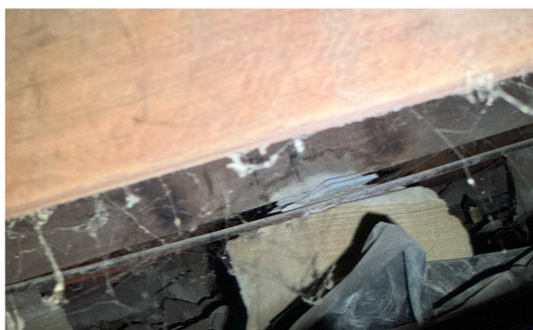
Figure 22 - Evidence of prior packing
