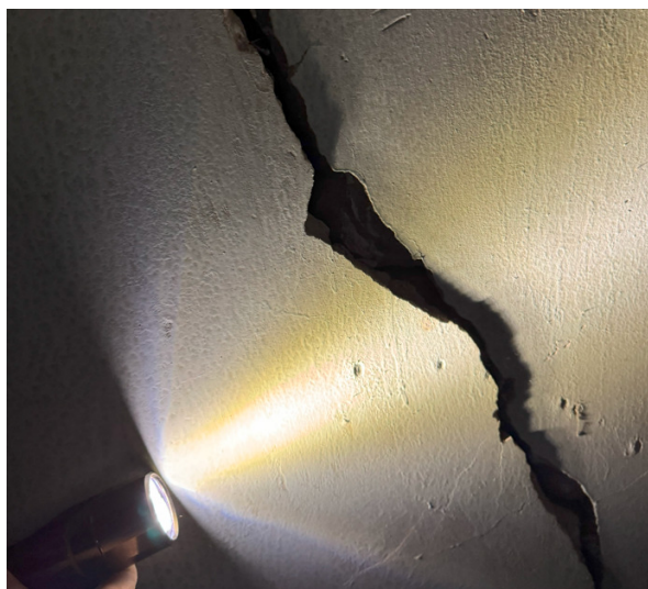
Figure 18 - Crack showing evidence of lateral movement of wall
