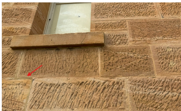
Figure 19 - Evidence of prior patching and replacement (external view)
