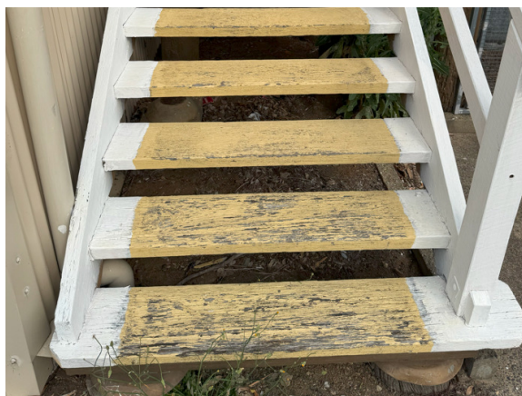
Figure 30 - Stair tread rot
