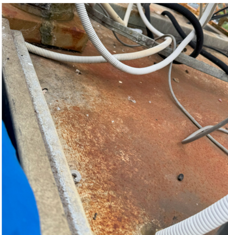
Figure 5 - Corrosion to flashing and pan
