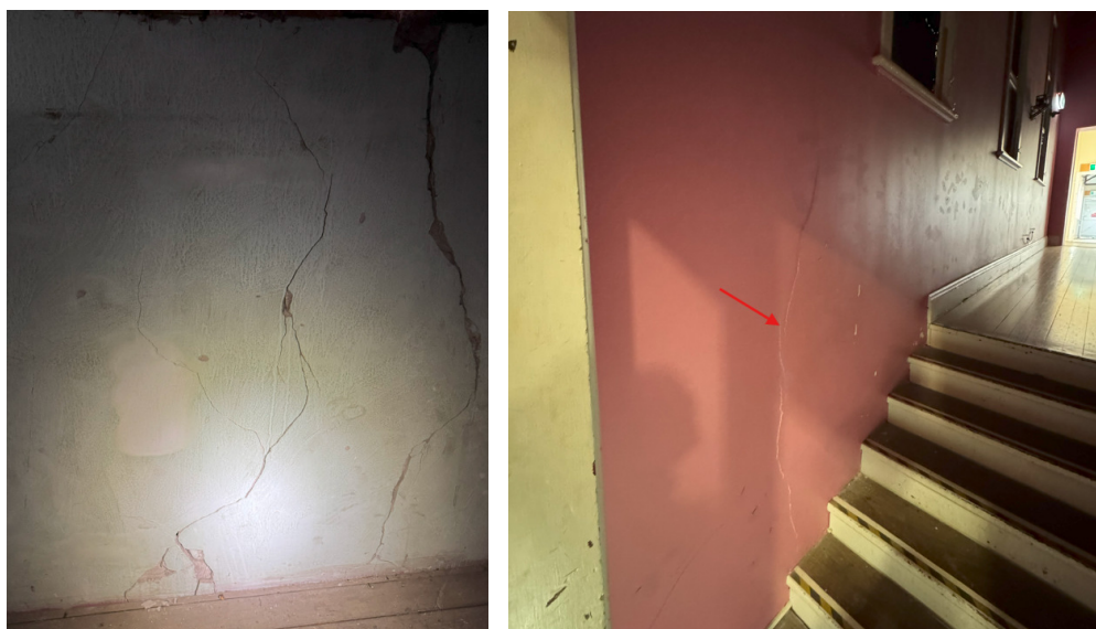
Figure 17 - Cracks to northern elevation at stage (internal view)
