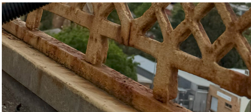
Figure 7 - Corrosion at base of balustrade
