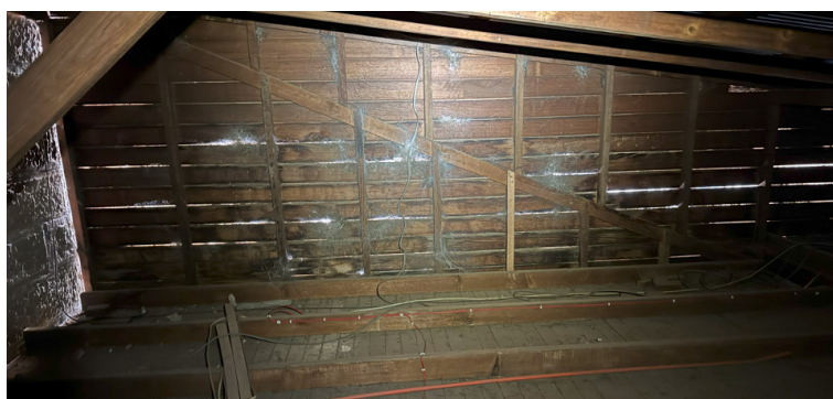
Figure 24 - Deteriorated Weatherboards (north elevation shown)
