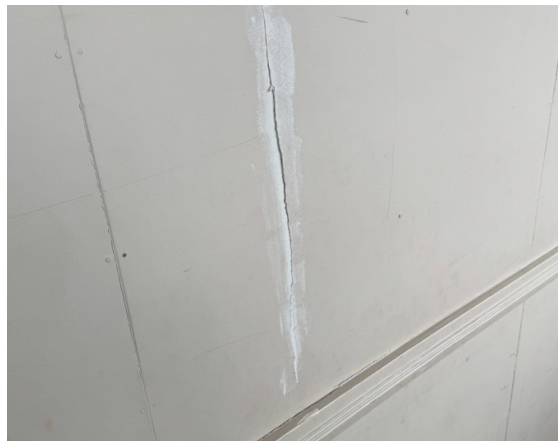
Figure 26 - Damaged internal lining
