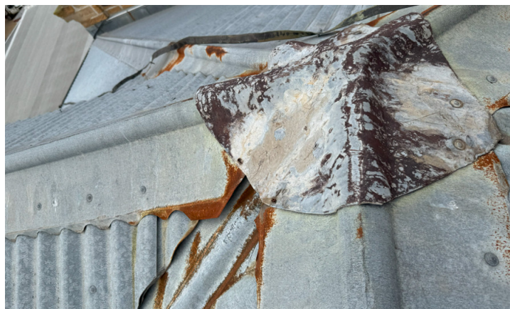
Figure 9 - Condition of capping and flashing above dormer
