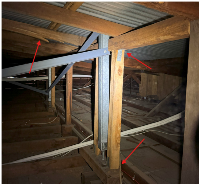
Figure 23 - Poorly propped roof beams and failed rafter
