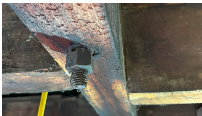
Figure 4 - Loose nut on flagpole hold down bolt
