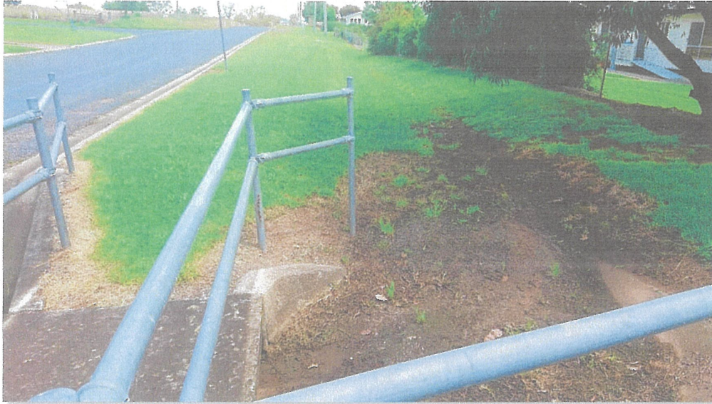
Figure 12 - Culvert outlet siltation
