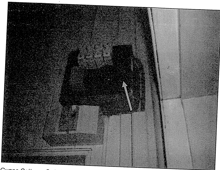
Gunns Cottage: Switchbox, ACM Resinous Backing Board & suspect internal ACM board
