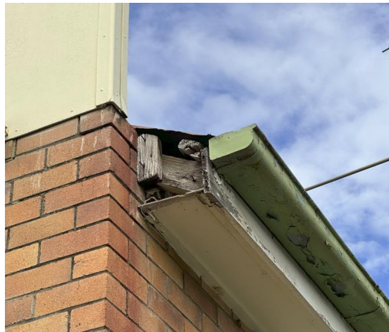
Figure 7 - Rot of Roof Framing Timbers where Exposed
