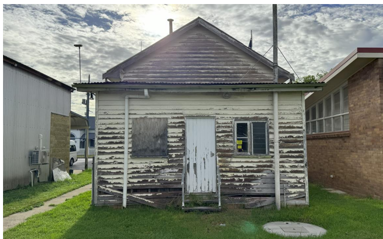
Figure 9 - General Cladding Deterioration and Loose Weatherboards
