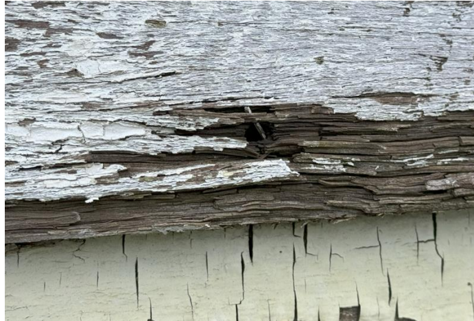
Figure 8 - Weatherboard Deterioration
