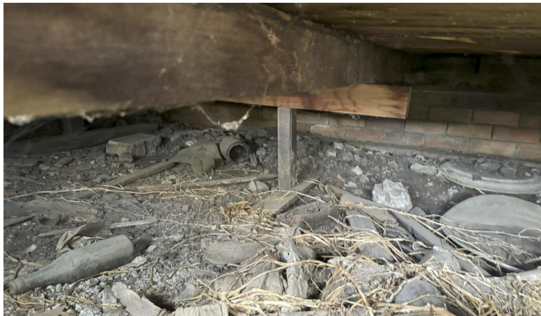
Figure 6 - Evidence of Previous Propping
