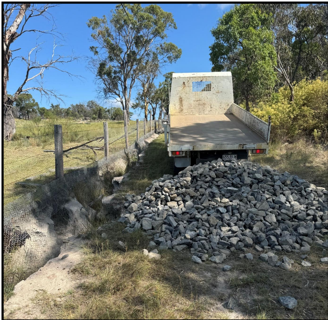
Plate 2. Shot rock being used to fill and stabilise the scour.
