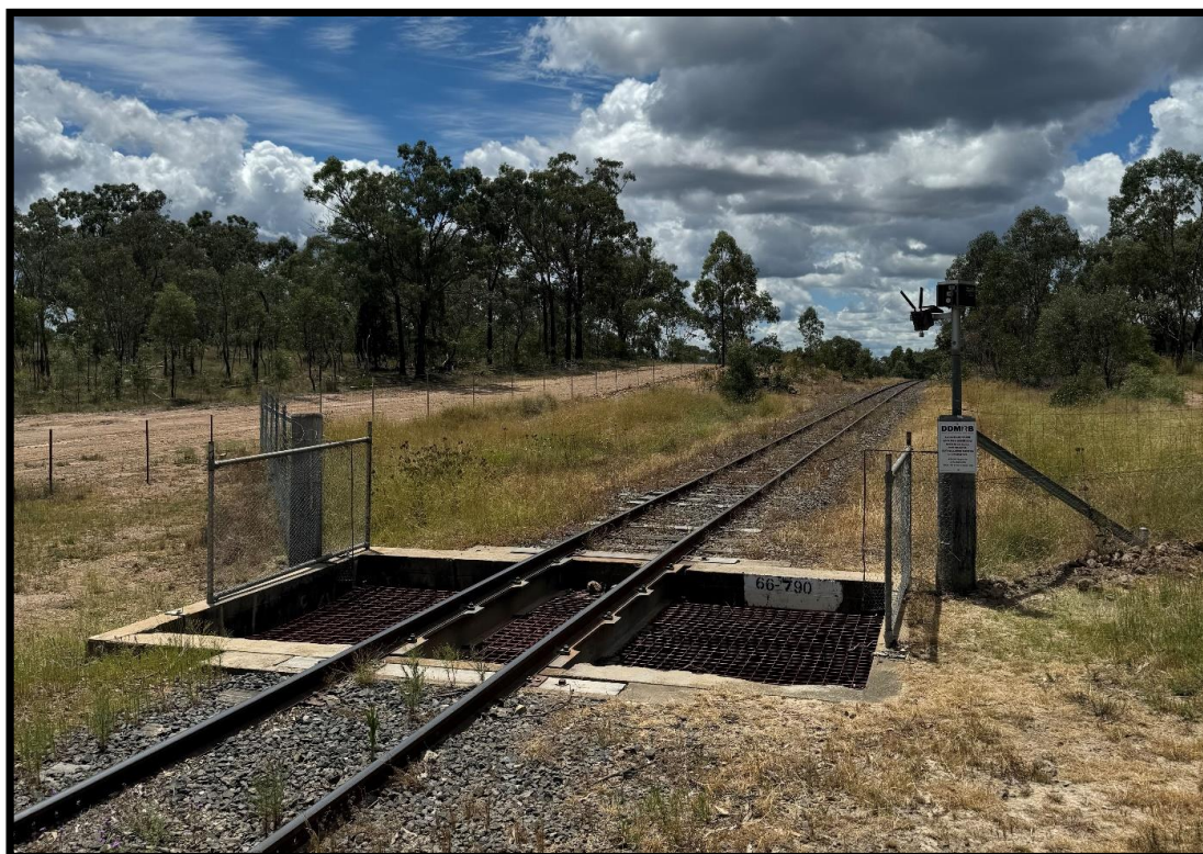
Plate 3. Siren and IR camera at QR inspection pit, Karara.
