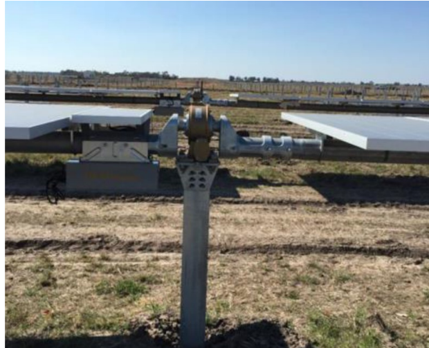
Figure 4 Proposed single axis tracker mount system
