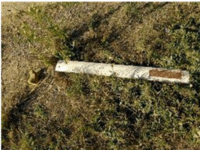
Exhibit 36. Guide post flattened by vehicle forced off the road.
