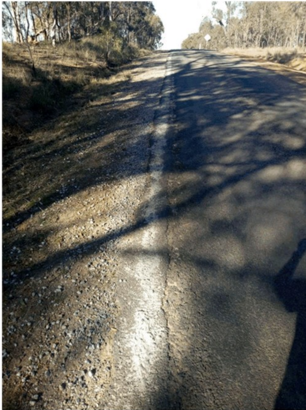
Exhibit 35. Narrow sealed section on Barlows Gate Rd is only one vehicle wide.
