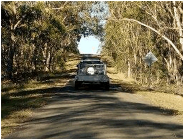
Exhibit 35. Narrow sealed section on Barlows Gate Rd is only one vehicle wide.
