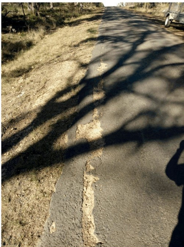
Exhibit 37. Repairs to the edge of the road rapidly degrade due the excessive heavy vehicle traffic.
