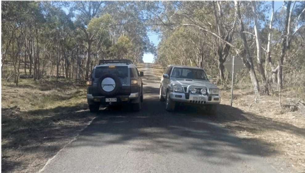
Exhibit 38. Two cars cannot pass on the sealed section of Barlows Gate Rd without driving off each side of the road.
